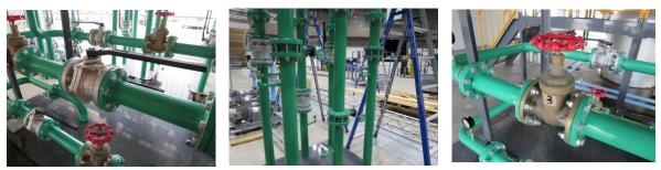
From left: Ball Valve, Rubber Seated Valve, Gate Valve
